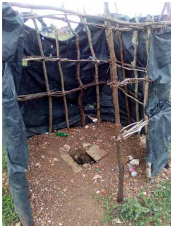
Pit latrine on a mine site in Shinyanga (2017 – Photo: IPIS)
