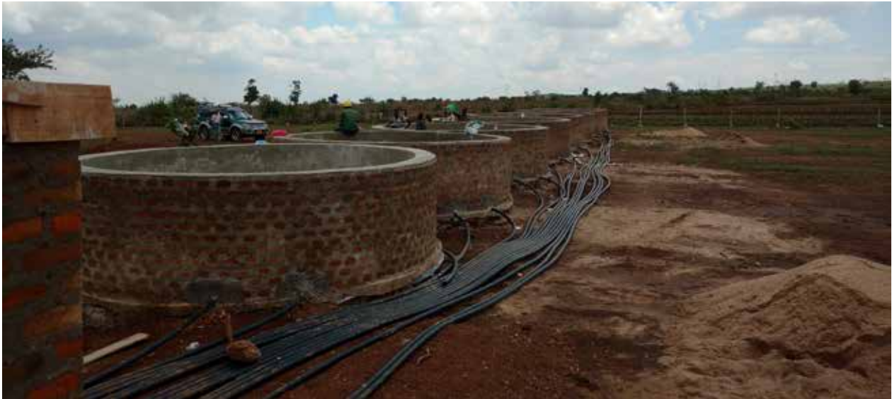
Cyanide leaching plant under construction (Mara, 2017 – Photo: IPIS)
