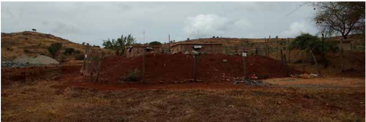
Pit shelters (1), Mining rush turning into a makeshift village with shops, guesthouses and restaurants (2), Permanent explosive storage building (3)
